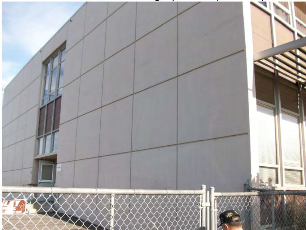
Photo 2: Exterior Side facing 8 th Street (West Side)
