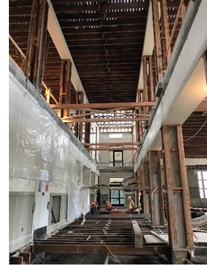
Old interior concrete 2 nd floor removed
