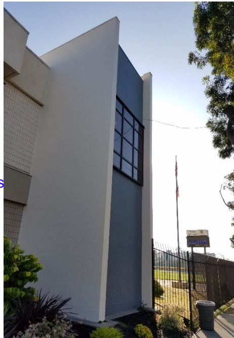
Top: Waterproofing/painting block walls due to winter rain, Alameda High
