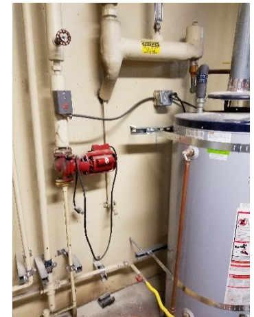
New water heater with earthquake strapping
