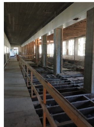
Demolished and ready for soil stabilization
