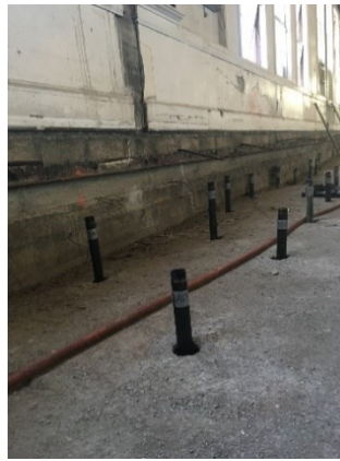
Grout injection, Interior
