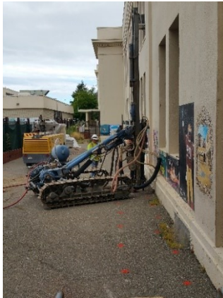
Grout injection, Exterior
