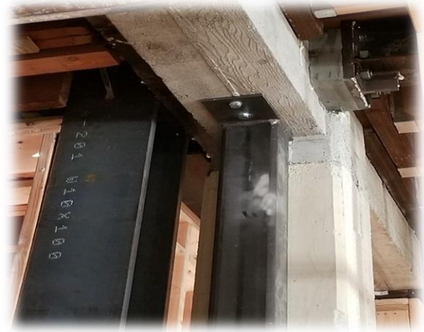
Structure Columns Repair
