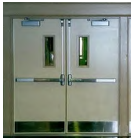
Panic Hardware on inside of exit doors
