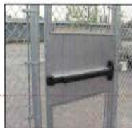
Gate with exit device for safe dispersal.
