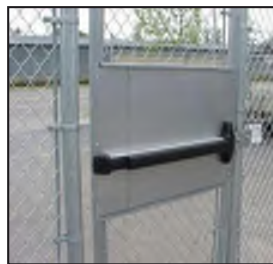
Gate with exit device for safe dispersal.
