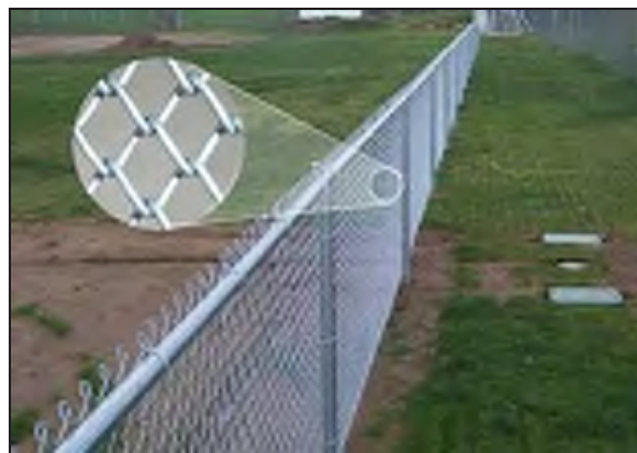
Chain link perimeter fencing
