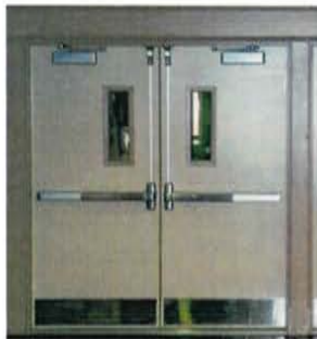
Panic Hardware on inside of exit doors
