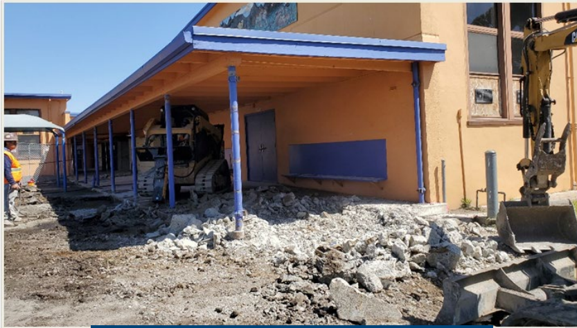
Demolition of concrete ramp
